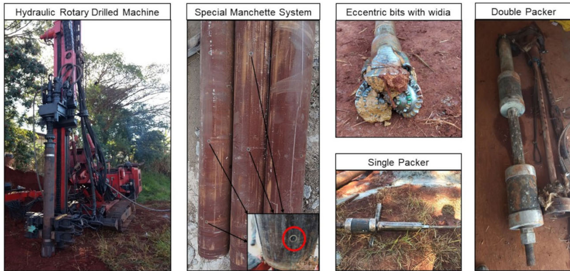
Fig. 3 Main features used during the micropiles installation
