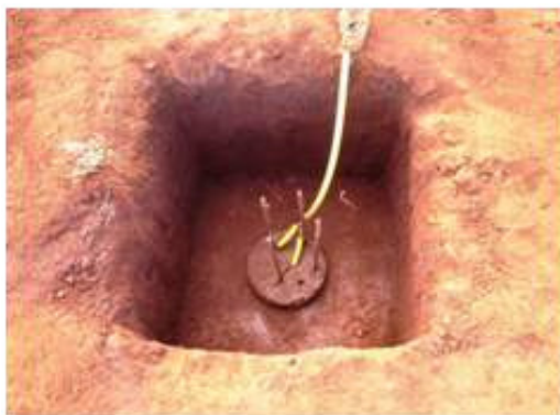
Figure 7 Excavation to the leveling mark of the pile for DPR_{(EXP)} .
