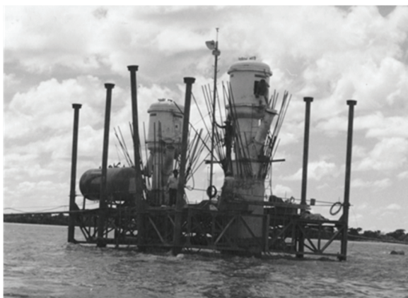
Figure 5. Example of pressurized drilled caisson platform and work site over a river in Brazil
