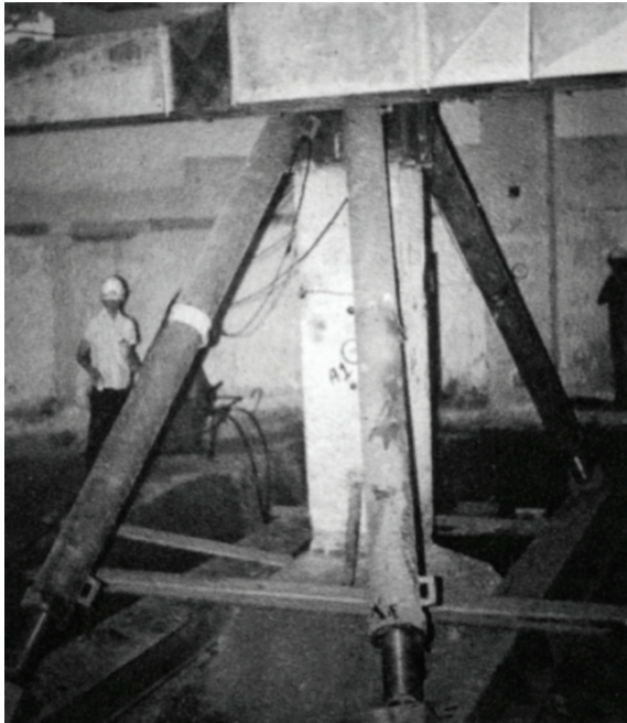
Figure 7. Foundation reinforcement at Paulista Mall ([2])
