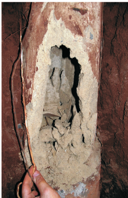
Figure 21 - Detail of the defect after performing the load test on block CD_{(EXP)} .
