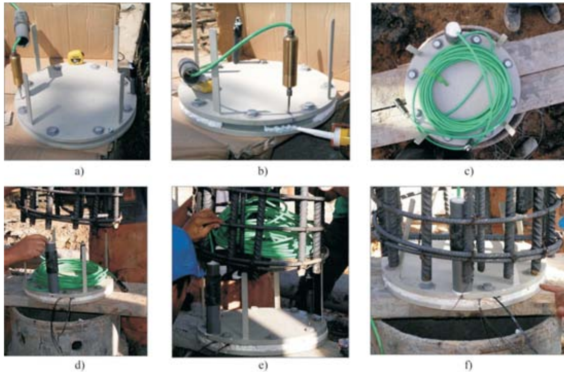
Figure 14 - Load cell installation (Costa Esteves, 2005).
