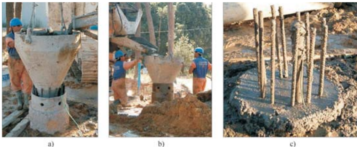
Figure 11 - a) and b) Piles concreting; c) Finalized concreting (Costa Esteves, 2005).
