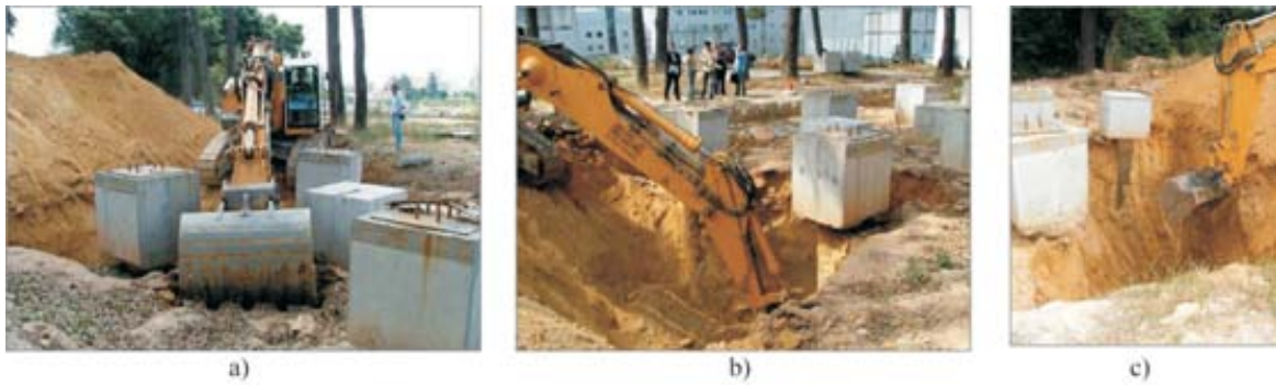
Figure 19 - Excavation: a) beginning of job; b) c) steps for soil removal (Costa Esteves, 2005).
