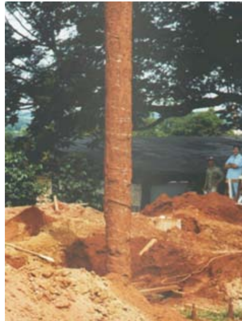
Figure 30 - Soil adherence in shaft of Omega 2 pile.
