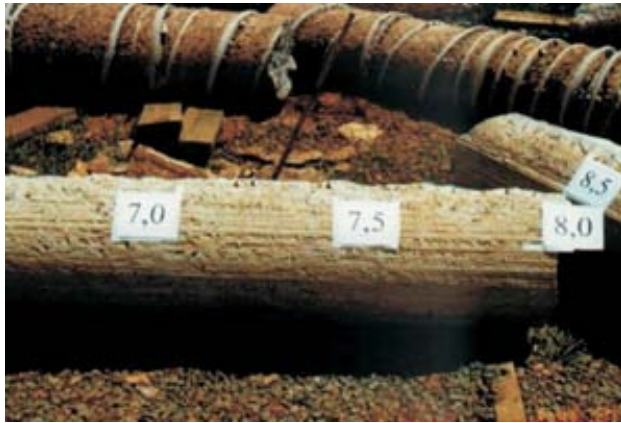
Figure 27 - Shaft view in CFA 2 pile (1 st plan).
