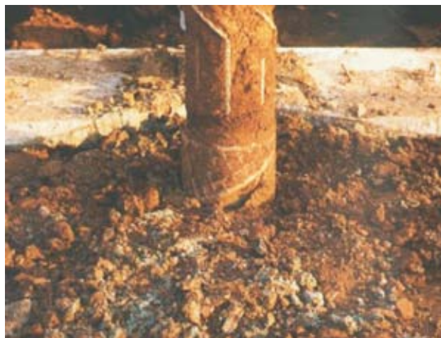
Figure 15 - Omega pile drilling.
