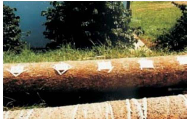
Figure 25 - Shaft view in bored 1 pile (2 nd plan) and in Omega 2 pile (1 st plan).
