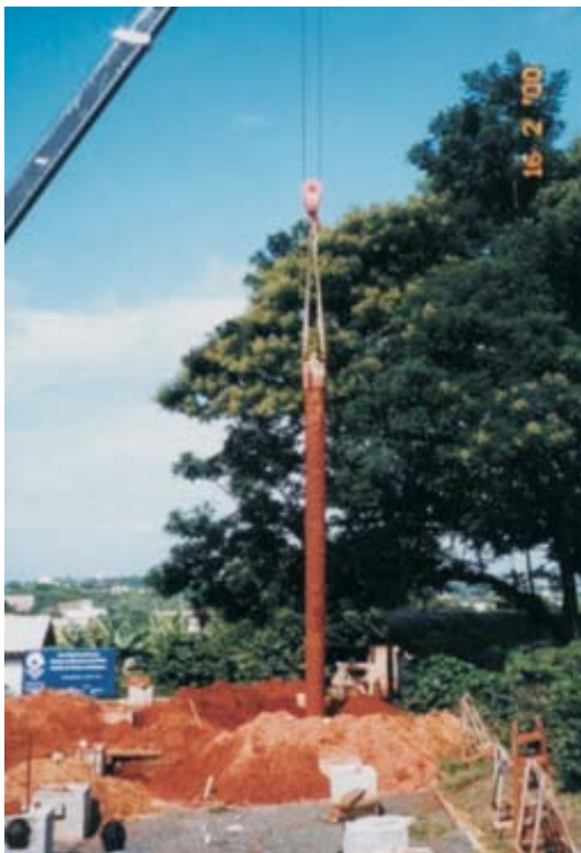
Figure 23 - Pile extraction.
