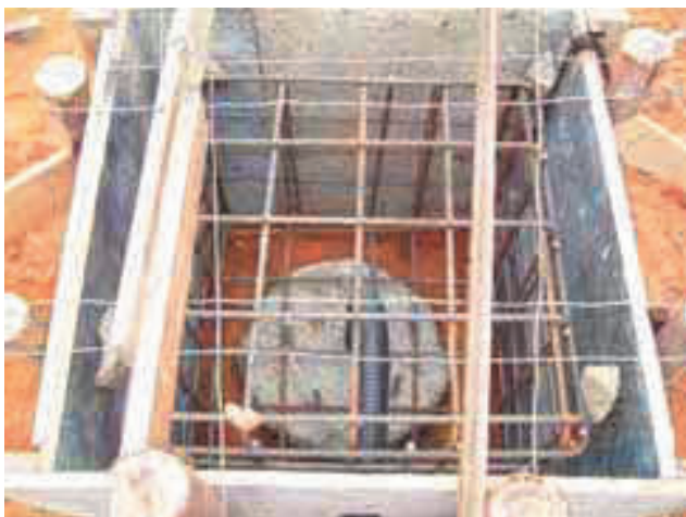
Fig. 20. Preparing the crowning block.
