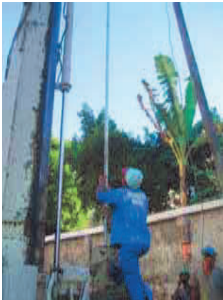
Fig. 16. Tube being placed in the pile
