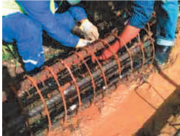
Fig. 15. Fastening the instrumented bar in the pile reinforcing cage
