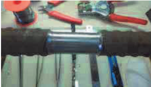
Fig. 9. Preparing the steel bar surface
