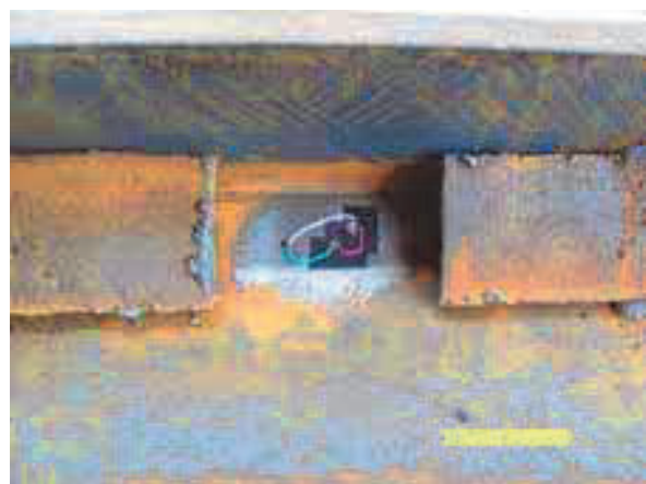
Fig 23. Strain gage fastened to the surface
